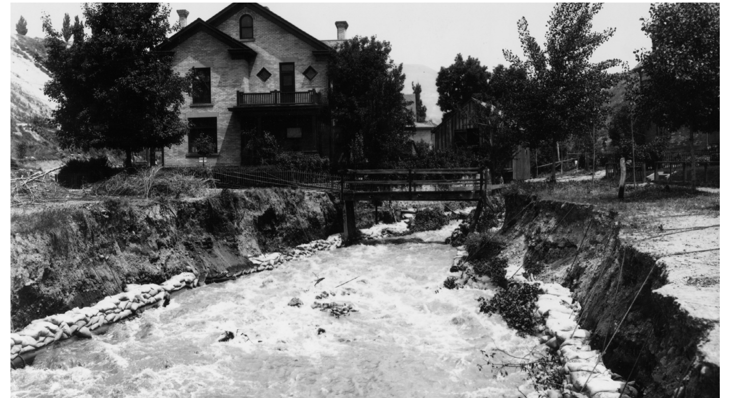
Figure 12: Banks of City Creek eroding near Canyon Road in Salt Lake City, circa 1909. Courtesy of Utah State Historical Society.
